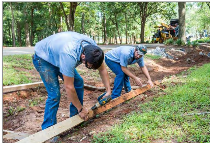
Construction of sidewalk for Community Safety & Mobility
