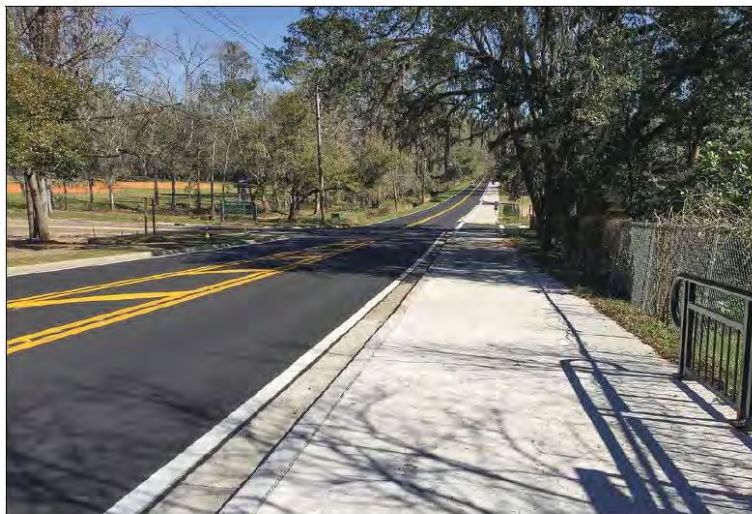
Local Road Resurfacing
