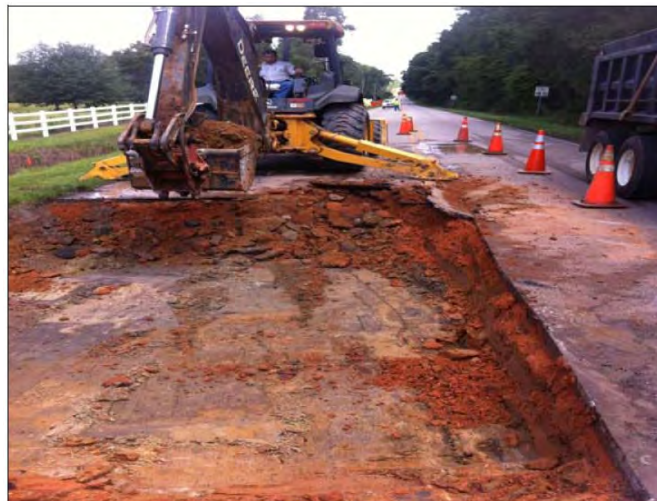
Asphalt Road Maintenance
