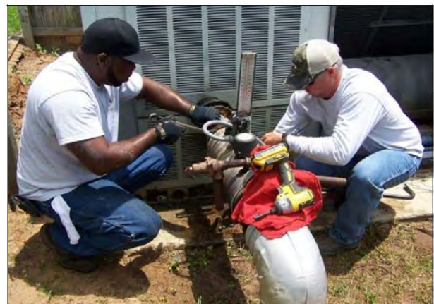
Building Mechanical Repairs and Improvements
