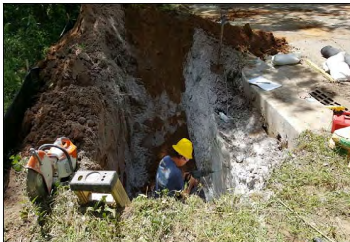
Stormwater Infrastructure Preventive Maintenance
