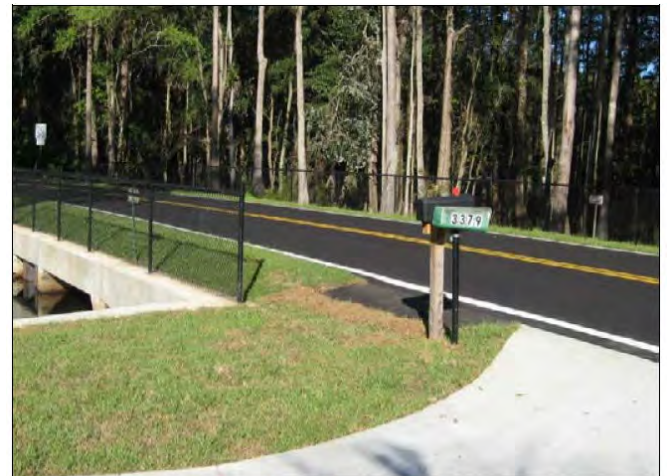
Private Road Paving
