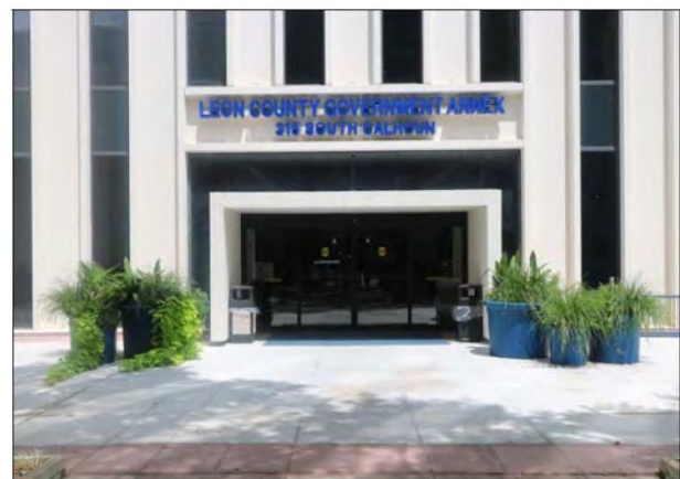
Leon County Government Annex Building
