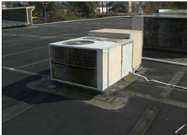
Building Roofing Repairs and Replacement
